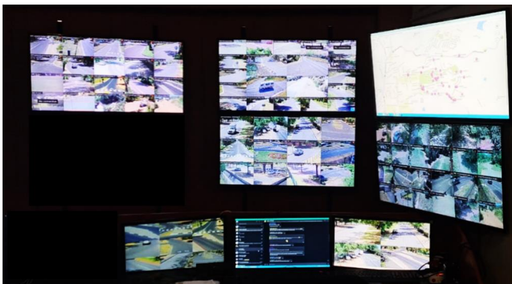
View of the monitoring screens in the JSRA Control Room
