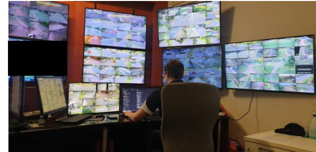
View of the monitoring screens in the JSRA Control Room
